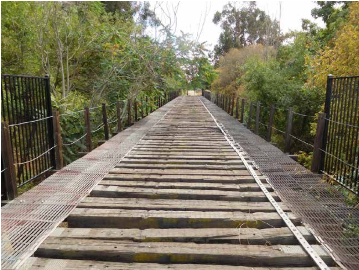
Photo 4: CA_Santa Clara County_Willow Glen Trestle_0004.tif
