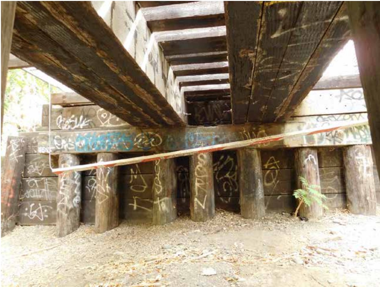
Photo 7: CA_Santa Clara County_Willow Glen Trestle_0007.tif
