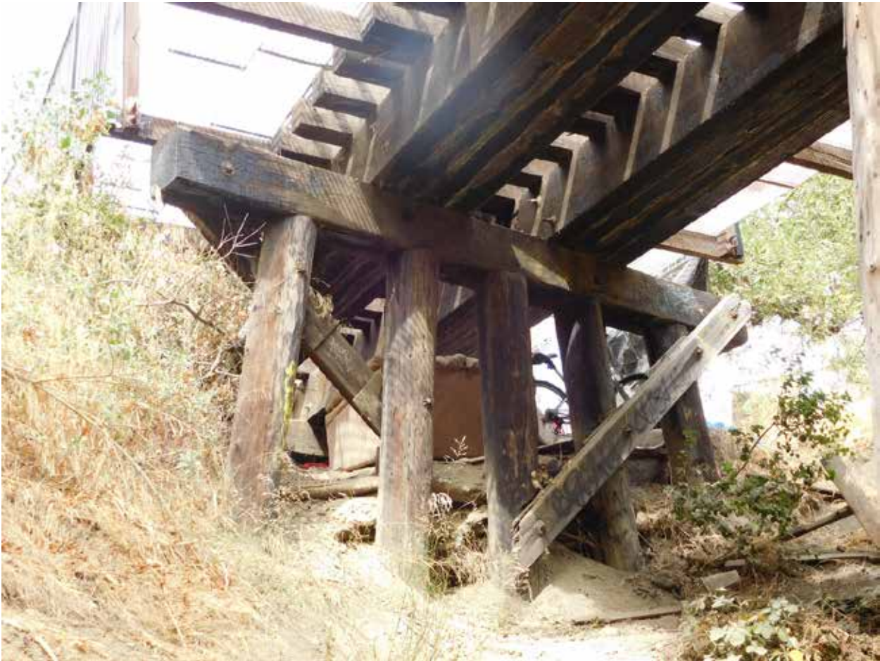
Photo 6: CA_Santa Clara County_Willow Glen Trestle_0006.tif
