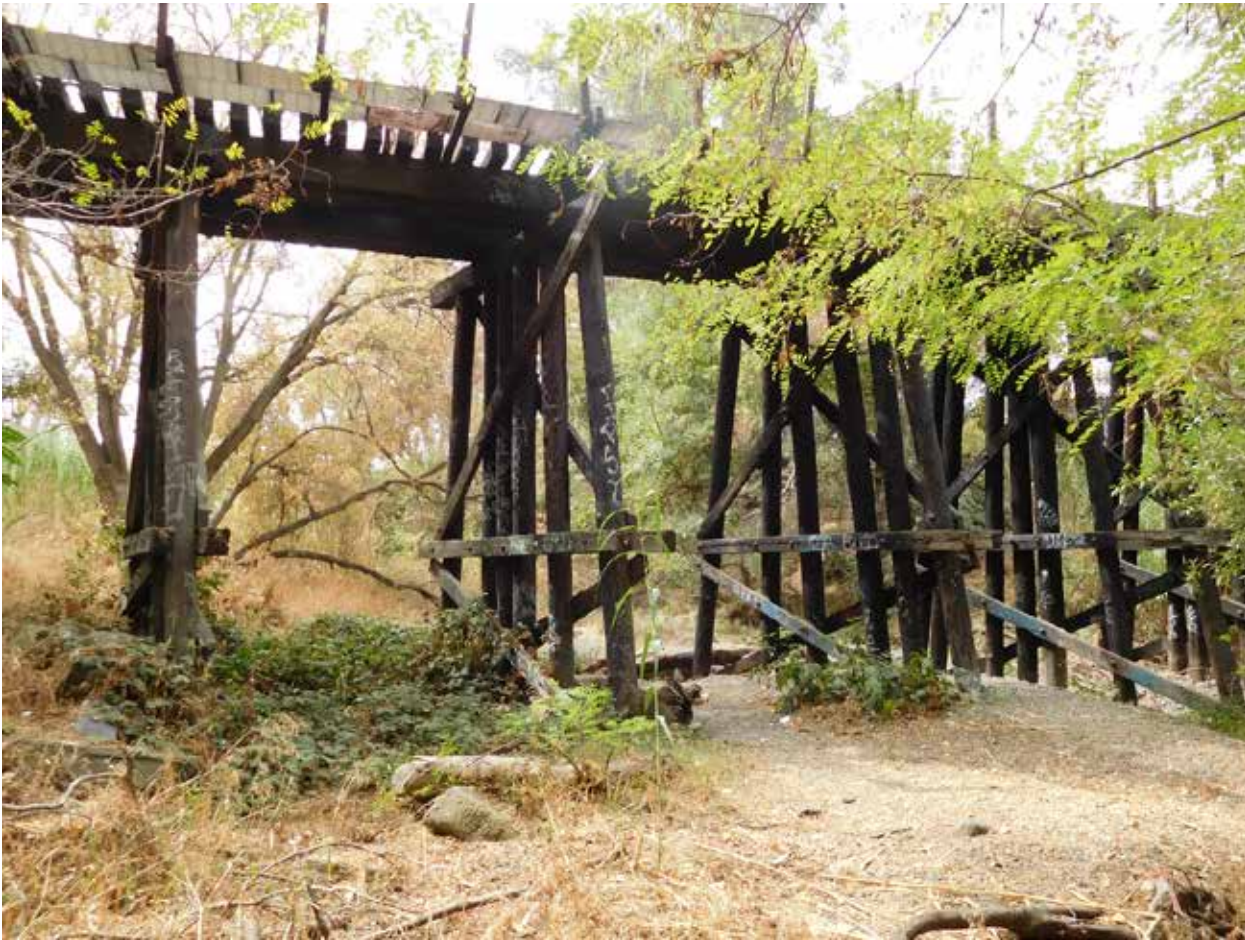
Photo 1: CA_Santa Clara County_Willow Glen Trestle_0001.tif
