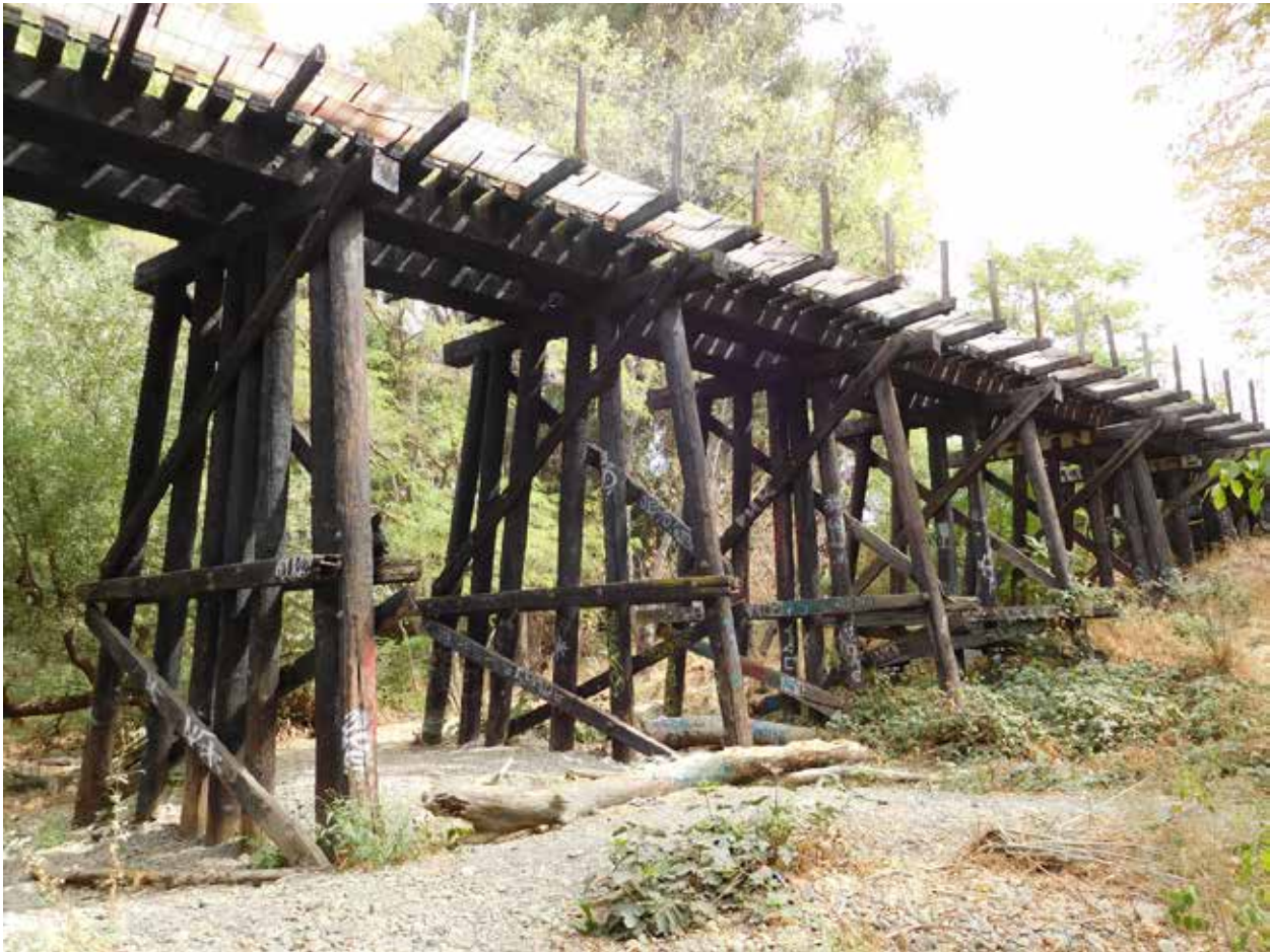
Photo 3: CA_Santa Clara County_Willow Glen Trestle_0003.tif
