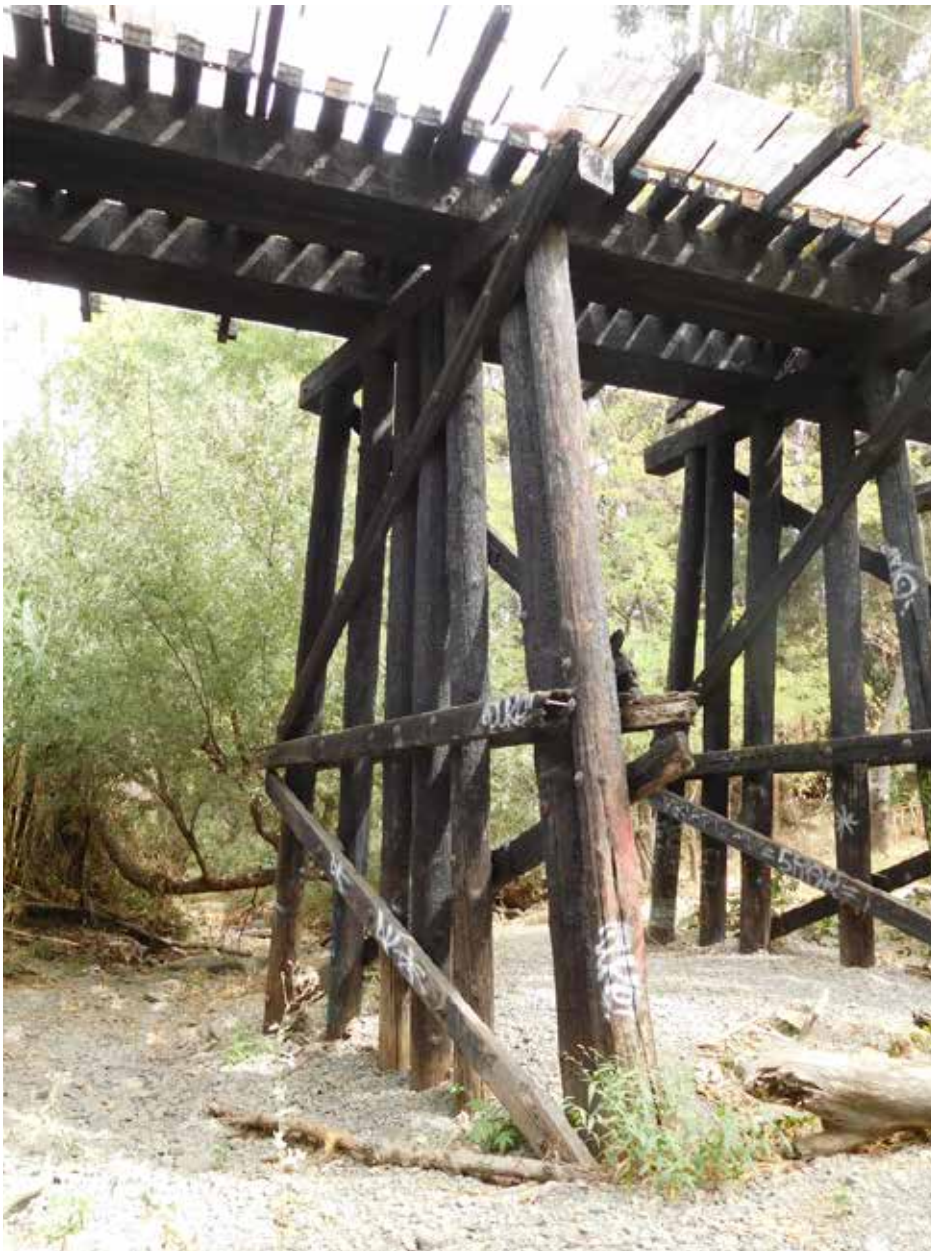
Photo 11: CA_Santa Clara County_Willow Glen Trestle_0011.tif
